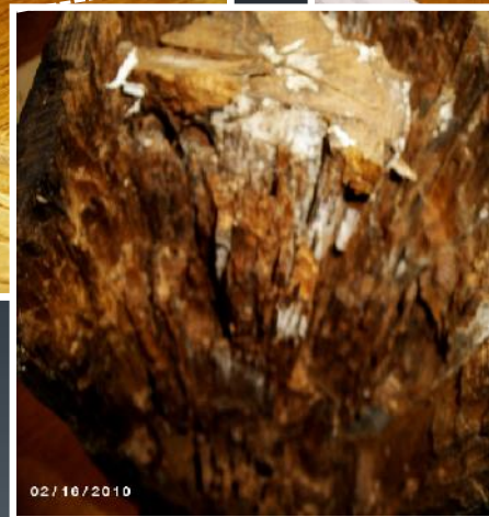
Rotted main support beams from Gym II
